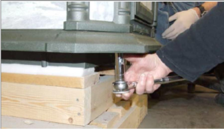
4. Locate the four Allen nuts that fasten the cast window frame front to the stove. There are two on each side of the frame.
